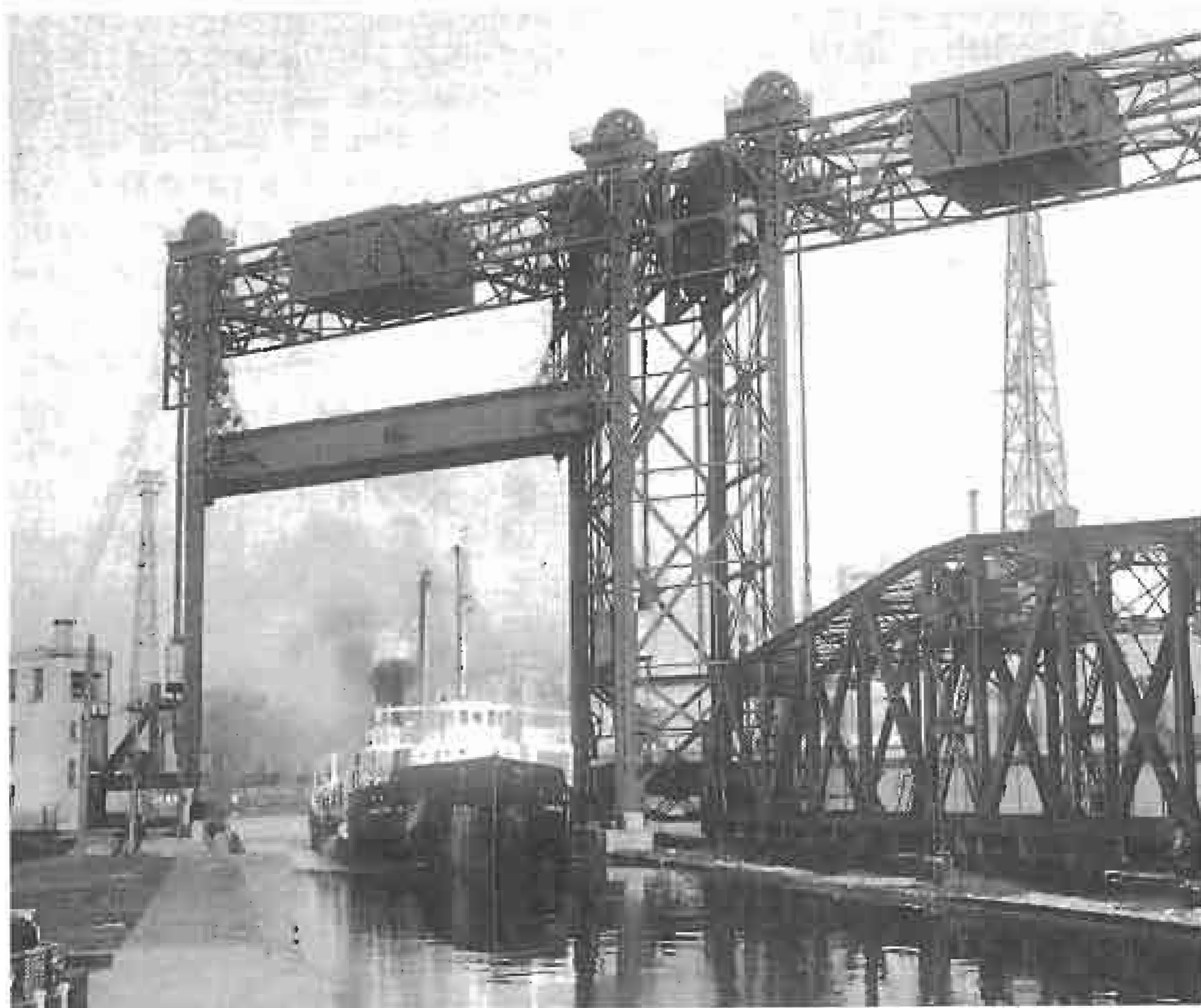
Rail traffic to and from Central Station comes to a stop at Wellington Interlocking Tower as switches and signals are locked favouring the passage of laker "Shelter Bay" under one of two 80-foot long lift spans which has been raised to a height of 90 feet over the Lachine Canal. The Tower is to the left of the photograph. The railway swing bridge at right serves local industry.
