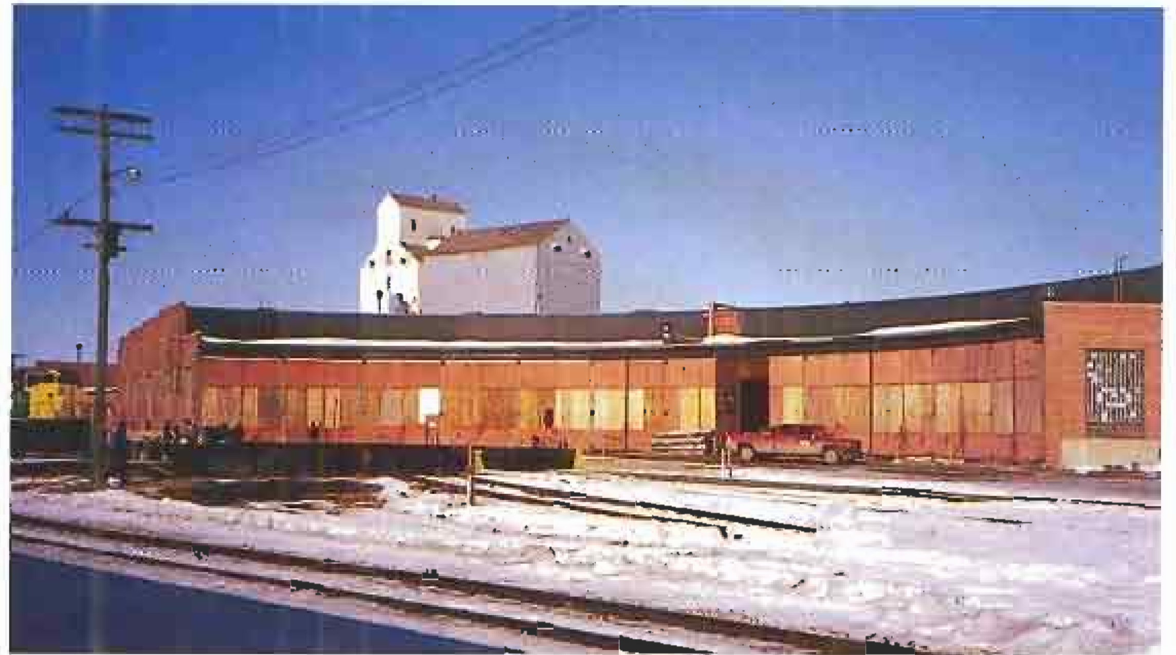
Canada's newest roundhouse, located in Prince Albert, Saskatchewan, was still active on February 26, 2000. Photo by George Gazuk.
