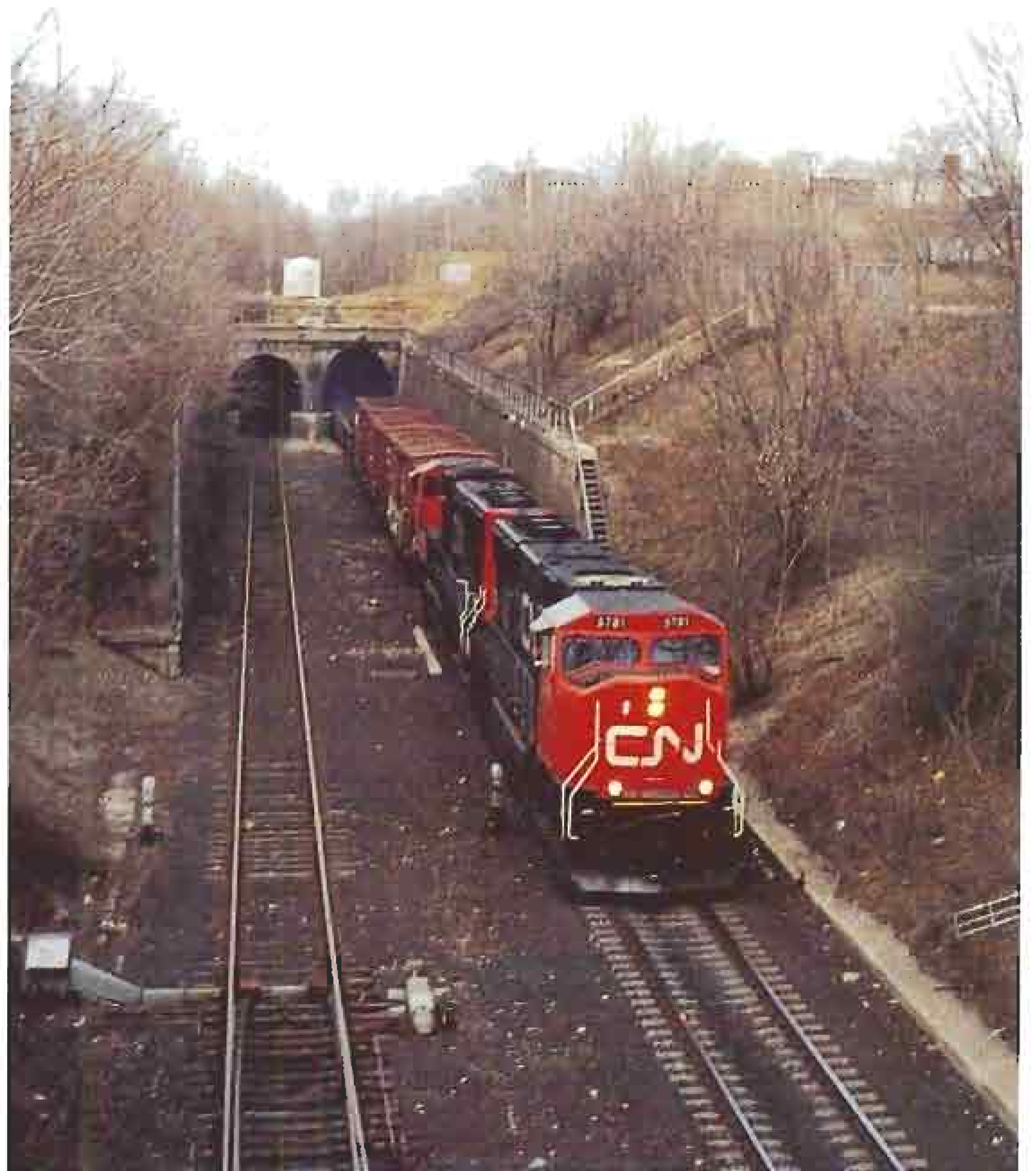
Bound for Windsor (Van de Water) Yard, a CN freight headed by SD751 5781 bursts from the enlarged north bore of the Detroit River Tunnel on February 26, 2000.
