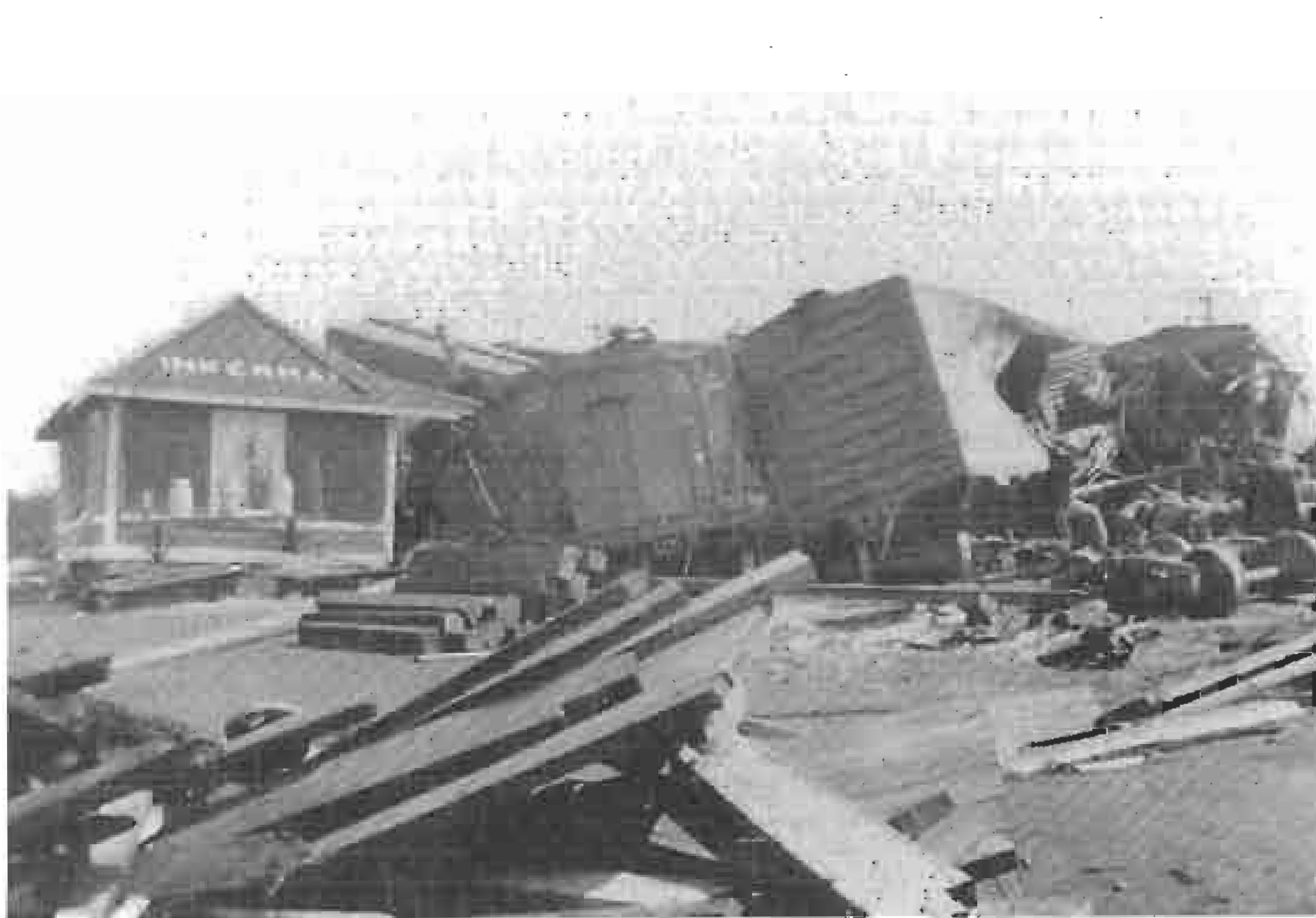
The Inkerman station survived, but barely, in fact it got physically moved north by about 3 feet. Notice the milk cans standing on the platform cart beside the building. No.29's engine is buried under those piled up box cars. Photograph: courtesy Mr. & Mrs. George Suffel.
