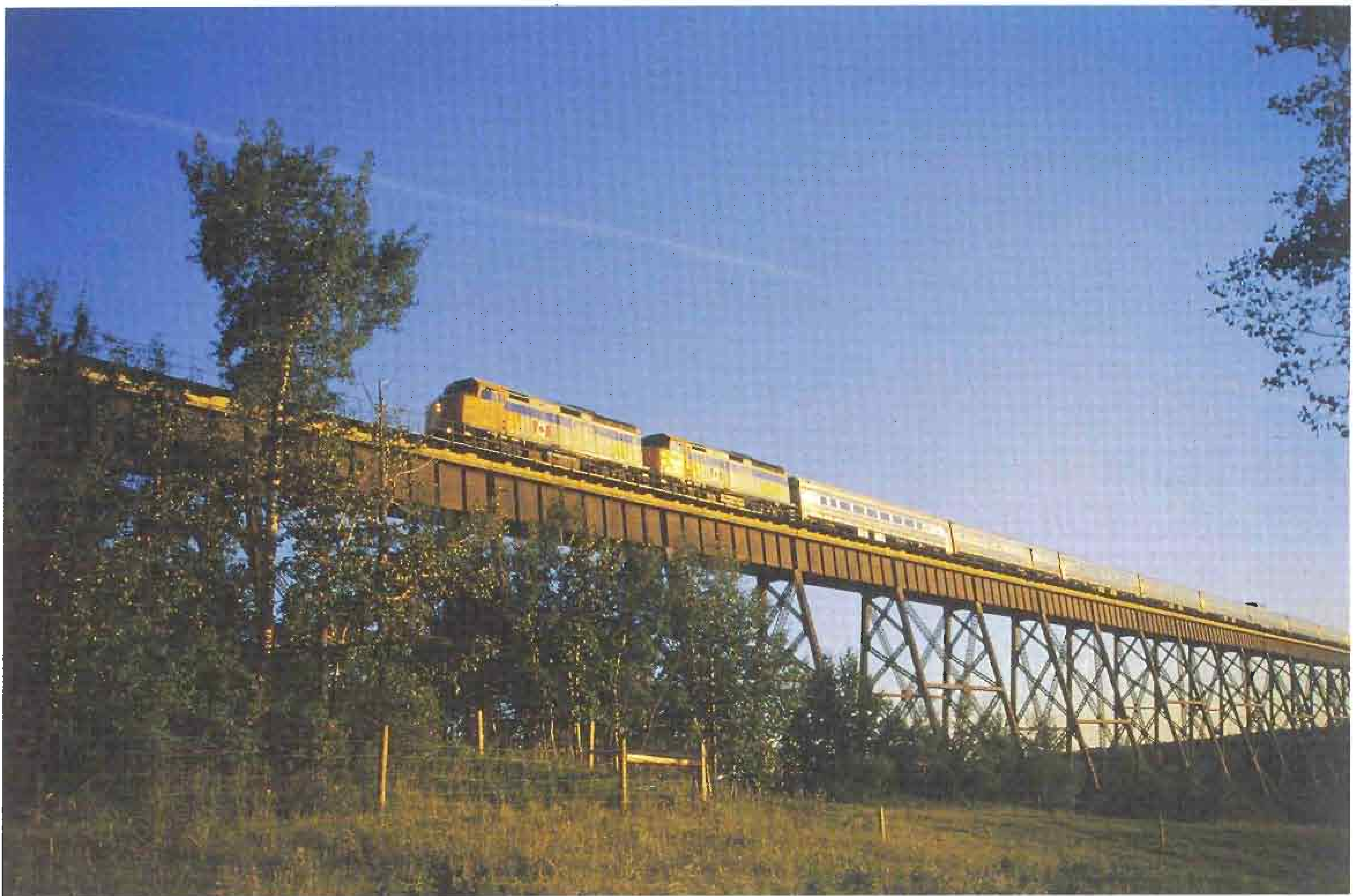
"In the Setting Sun" - Two VIA Rail F40PH-2 units lead the eastbound "Canadian" across the 2,775-foot long, 195-foot high trestle at Fabyan, Alberta, at 20:45 hours on July 23, 2001. The trestle is located at Mile 148 of CN's Wainwright Subdivision. Photo by Barry Williams.
