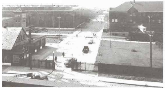
A view looking northwest from the Rachel Street gate. In the left foreground is the police office and fire hall. To the left of the midway is the locomotive erecting shop, while to the right is the general office building. To the right is a 6900-series 0-8-0 switcher. Photo courtesy of Canadian Pacific, from the author's collection.
