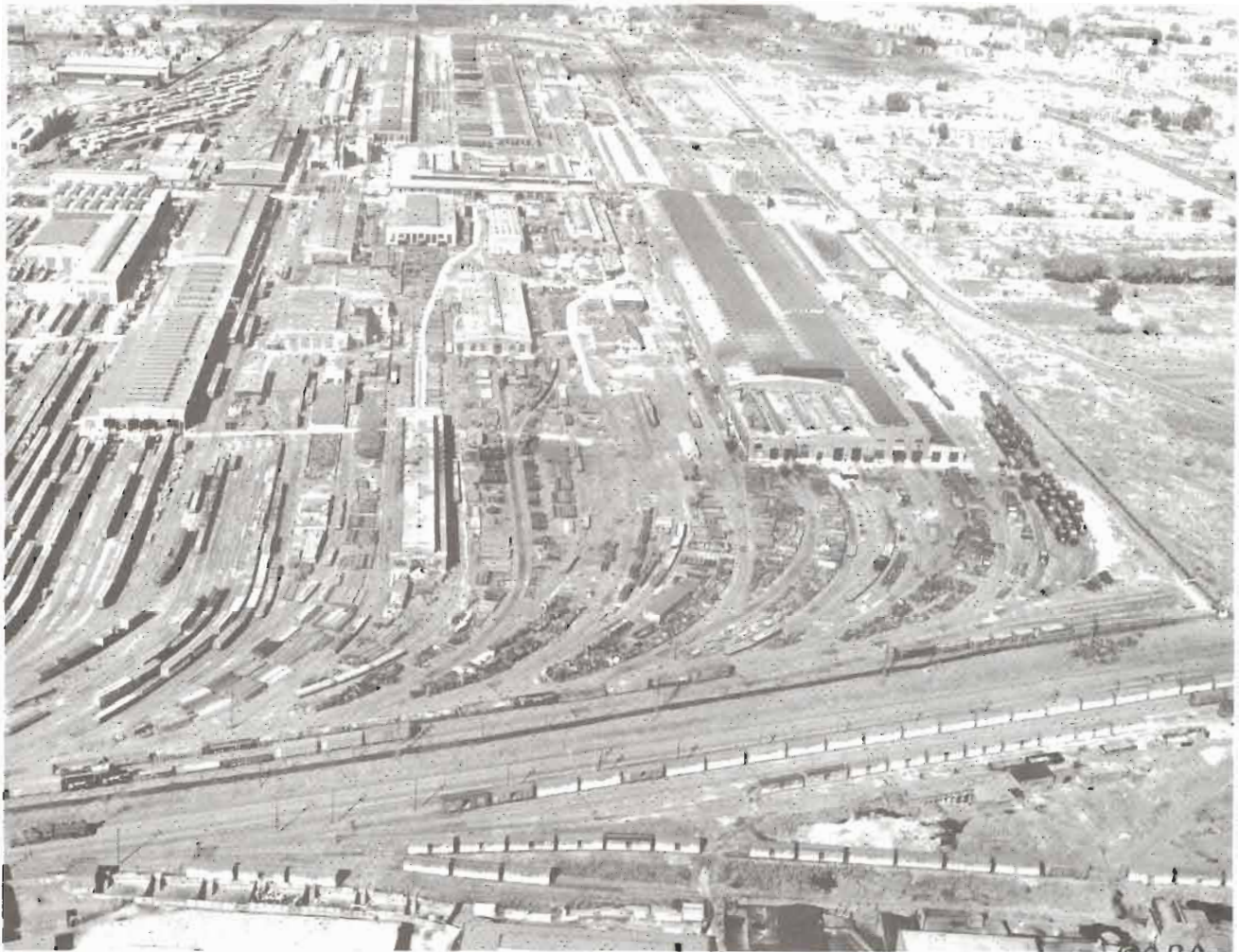
Angus Shops as they appeared in July 1951. The photograph is taken facing geographic North, or, as the City of Montreal puts it, looks East along Rachel Street. Rachel Street runs from the bottom to top at the right side of the photo. Adjacent to it, the first large building is the locomotive erecting shop. Ancillary buildings come next, with the long freight car shop on the left hand side. Just beyond the locomotive and freight car shops lies the "midway" and beyond are the passenger car shops. Near the bottom of the photo a locomotive can be seen travelling on the main tracks of the Park Avenue Subdivision headed toward Hochelaga Yard and Place Viger. At the bottom are rows of stock cars on trackage of the Eastern Public Cattle Market, then a subsidiary of Canadian Pacific. (C.P. Archives photo, collection of the author)
