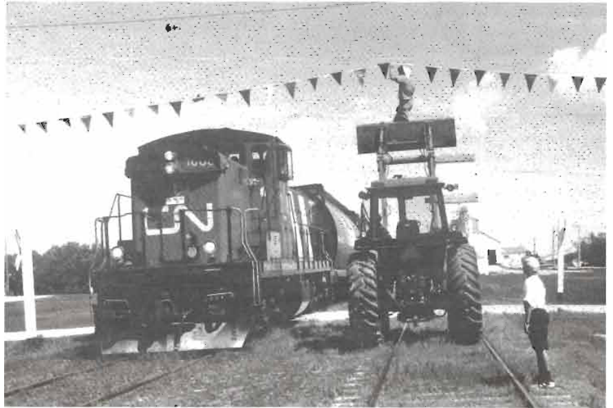
ABOVE: On July 25, 1996, GMD1u 1608 and the 14 cars of Train 549, with a little manual intervention, clear the 100 year reunion decorations at Fork River, Manitoba. LEFT: Weeds, cinders and ballast support aged ties and 56 lb. rail dating back to the beginning in 1896. This track is at Fork River on September 5, 1996. Both photos by Mark Perry.
