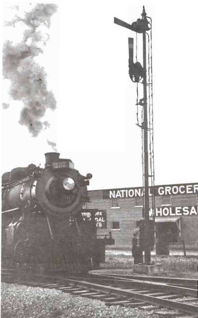
Mixed twice weekly T&NO No. 222 with Mikado No. 307 has arrived from Moosonee at the CN/T&NO crossing. With the lower arm semaphore set in its favour by the trainman, Train 222 will move over the crossing in this 1944 scene. The station is 0.44 miles ahead.
