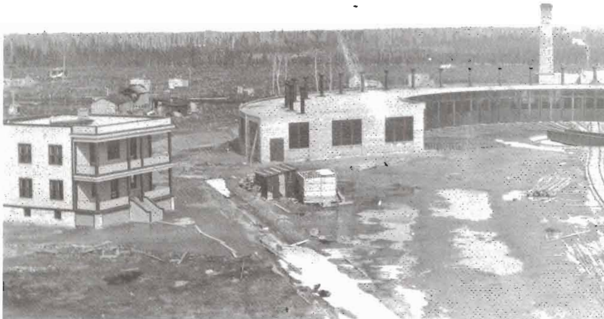
Just completed, circa 1918, Cochrane bunk house with offices for the locomotive and car foremen as well as the 18-stall roundhouse and machine shop. The locomotive facility was built to Grand Trunk Pacific plans.
