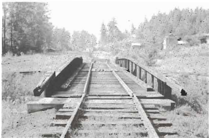
BELOW: The turntable at Arrowhead, British Columbia, on September 4, 1966. Within a couple of years, the whole site, including the town to the rear, would be under water.
