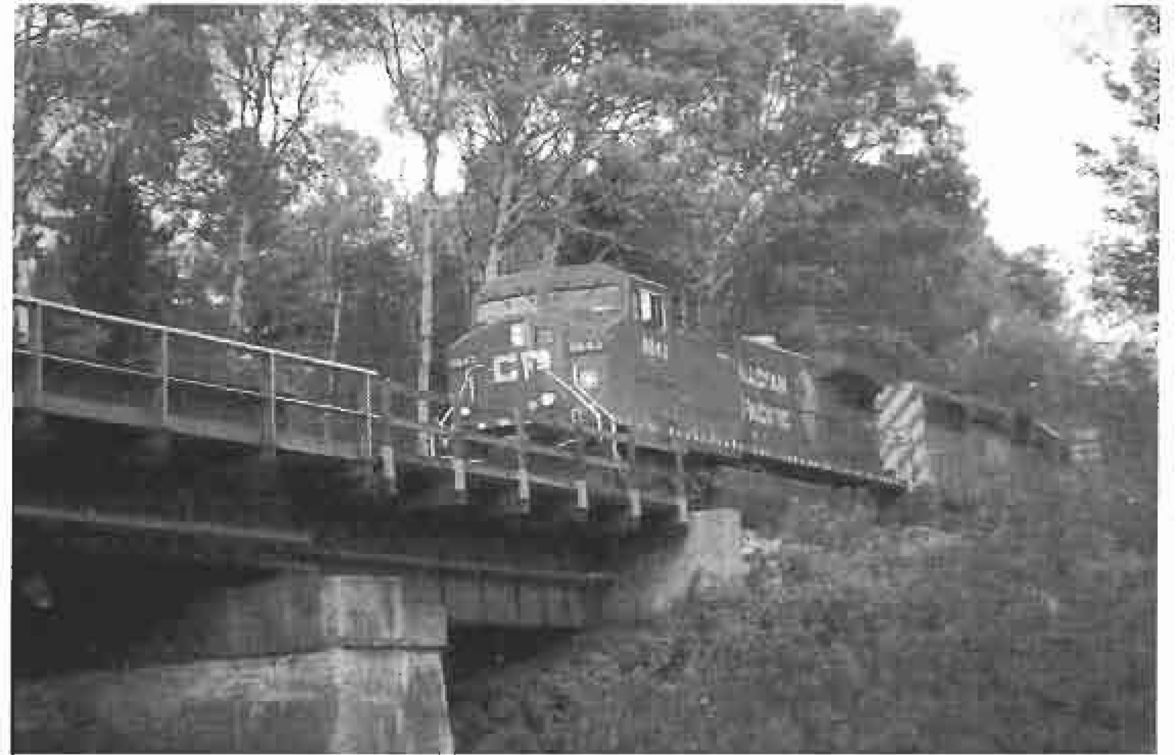
A CP southbound powered by AC4400CW 8643 and SD40-2 6026.
